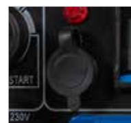
ATS panel connection
